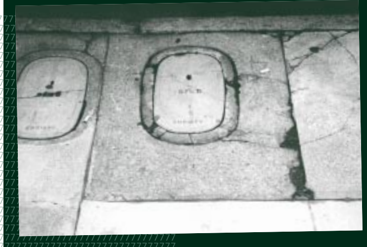
TWO SAN FRANCISCO WATER DEPARTMENT UTILITY PANELS IN TERRITORIES CHARACTERIZED BY EXTENSIVE TRANSFORMATIVE PROCESSES.
